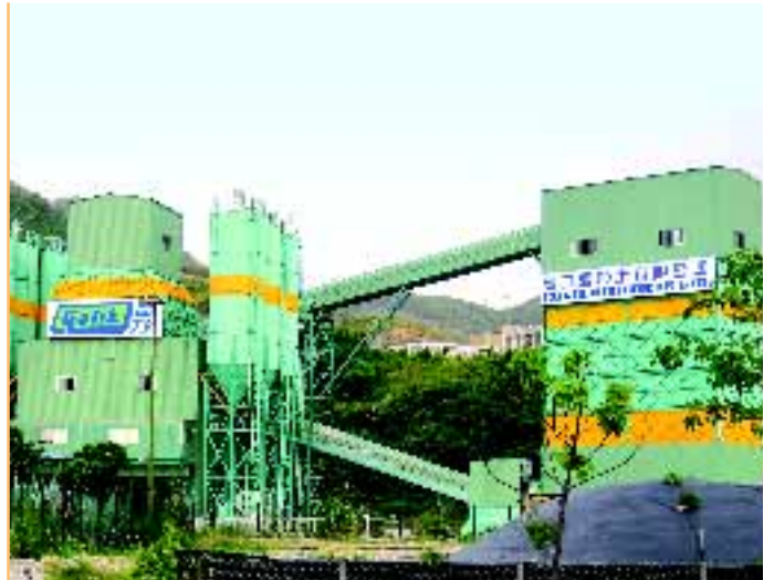
Ready Mixed Concrete Plant in Siu Ho Wan, Lantau, Hong Kong
