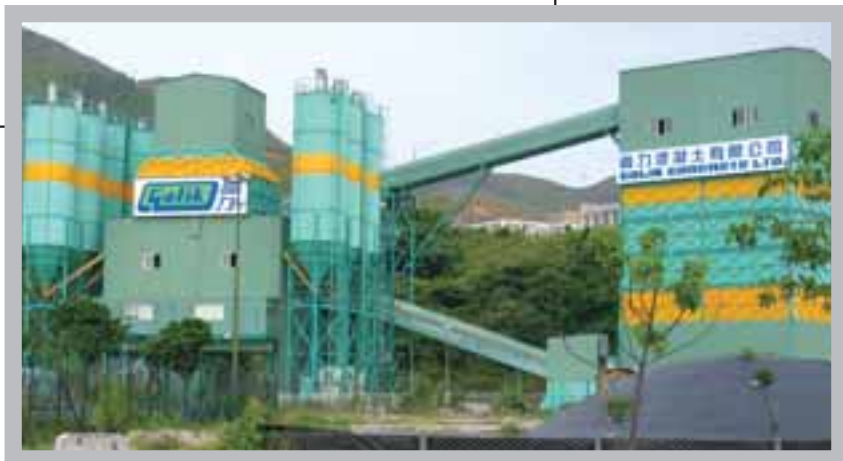
Ready Mixed Concrete Plant in Siu Ho Wan, Lantau Island, Hong Kong
